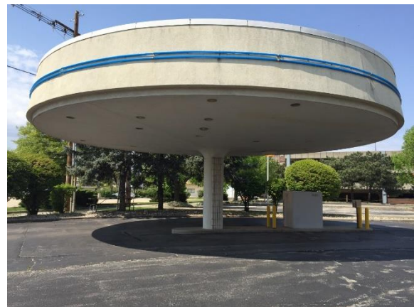
Figures 5 and 6. Images of a now defunct branch of the First Financial Bank of Danville, Illinois. The cantilevered drive-up service stations offer strong hints of radial organizations, imposing vertical and horizontal cantilevers, and the unseen strength of steel reinforcement in concrete. The hints of structural logic abound all around a student's world.
